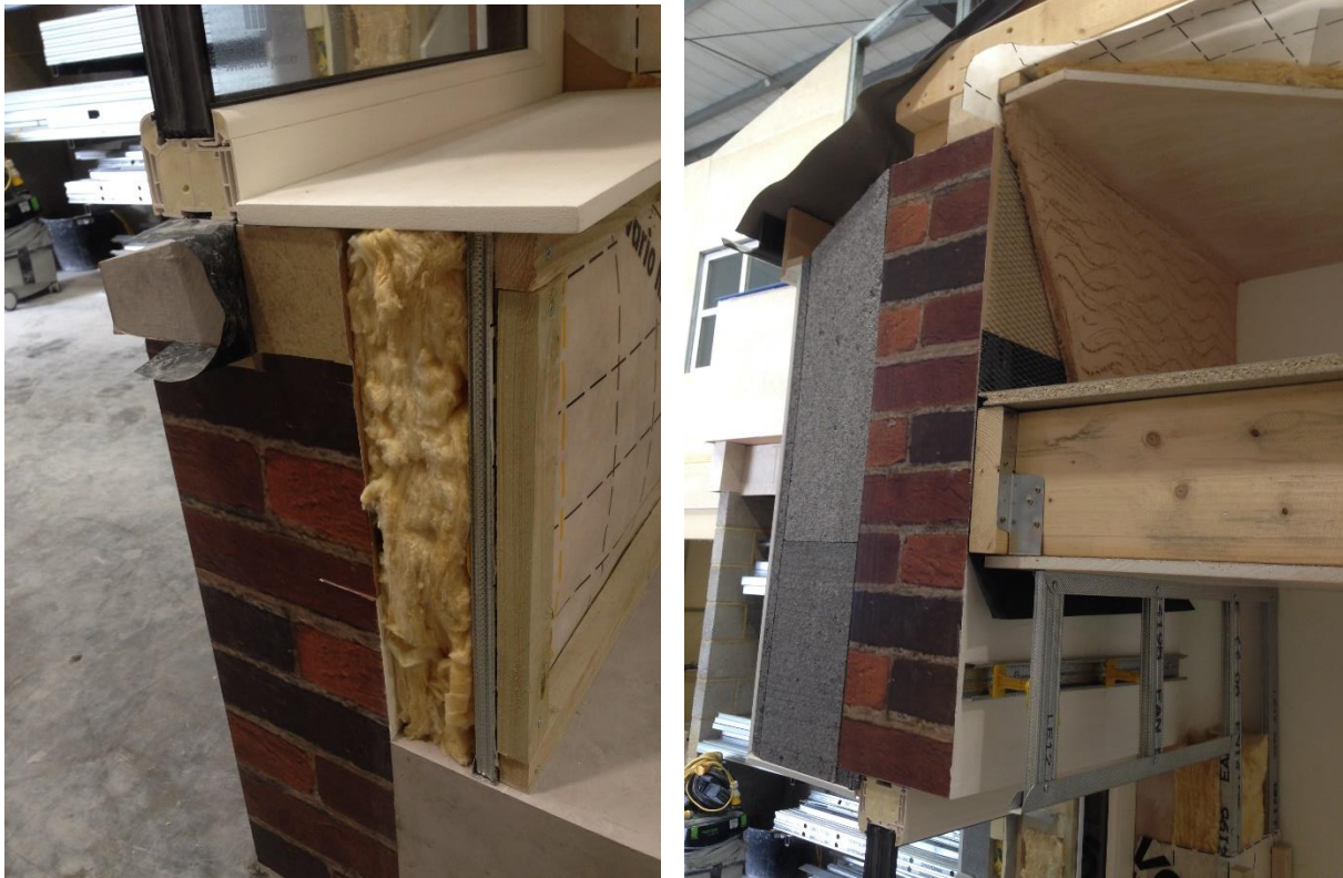
Figure 30: Images of brick external wall models internally insulated with rockwool (on the left) and externally insulated with polystyrene (on the right).
