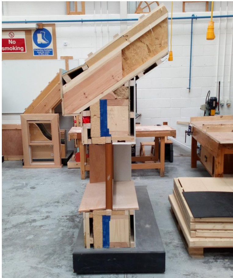
Figure 31: Timber frame model depicting retrofit of external insulation on wall and roof using wood fibre
