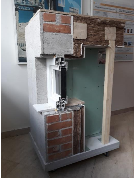
Figure 9: Model of the internal insulation on the existing masonry wall
