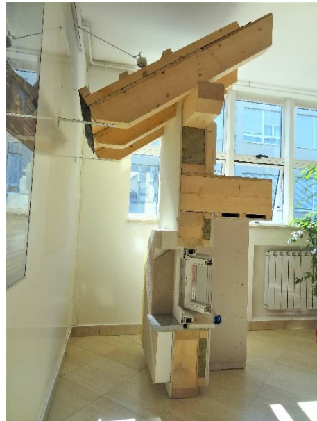
Figure 11: Model of the foundation detail (external insulation) and balcony detail (thermal break)
